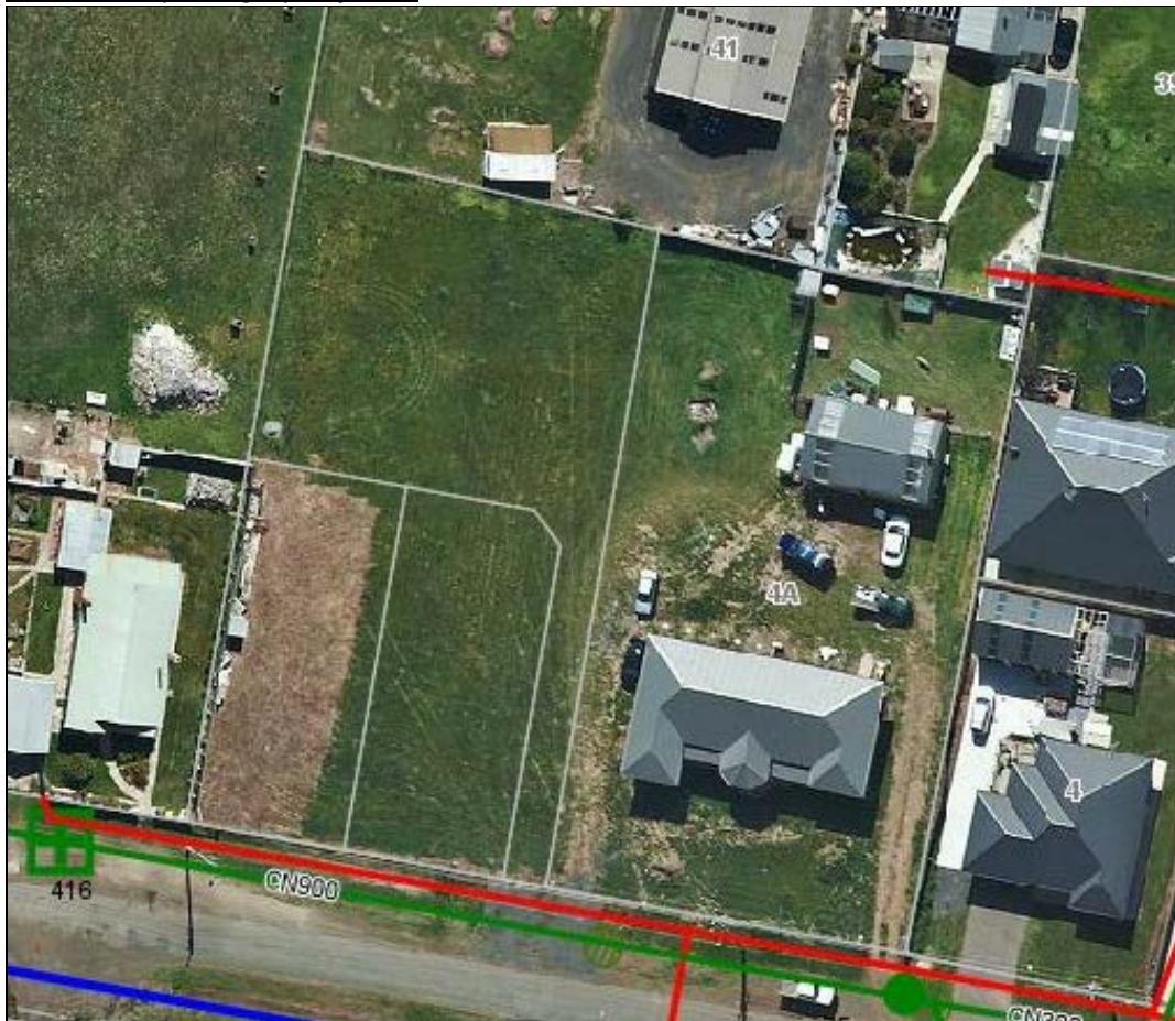
Photographs of subject site
