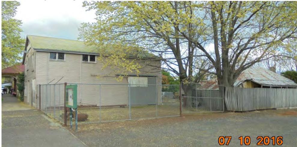
Subject site from High Street
