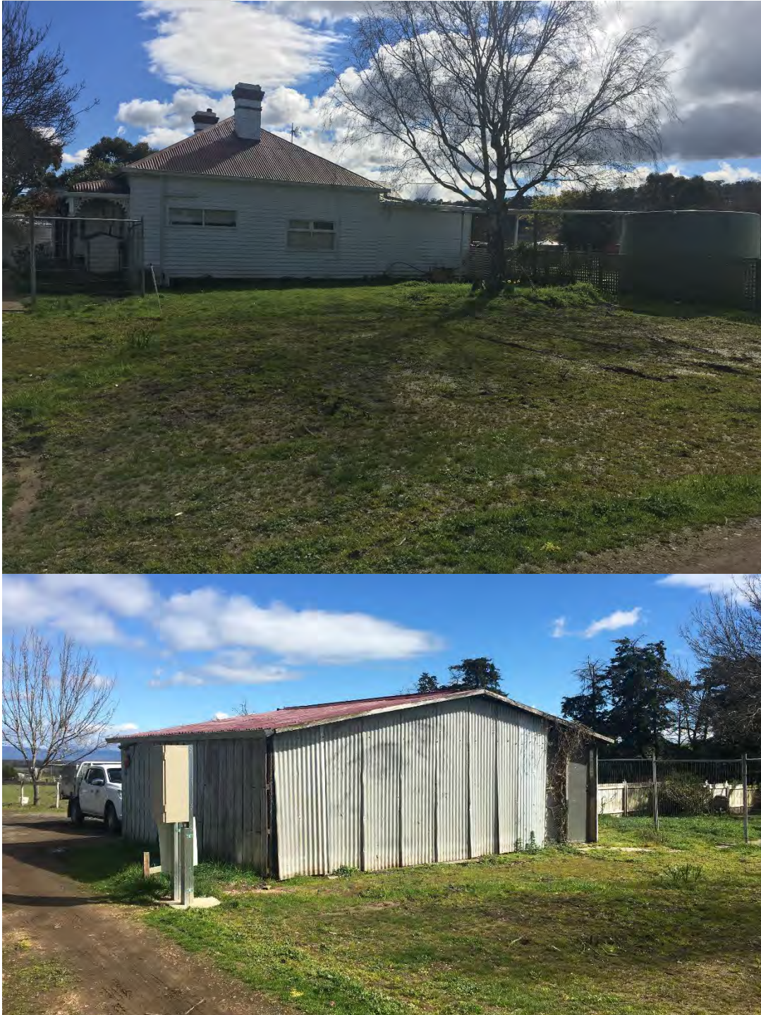
Photographs of subject site
