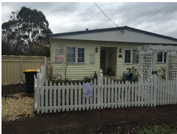
Photographs of subject site
