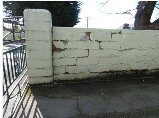
Wall to be replaced
