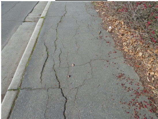
Footpath damage caused by Tree roots or sub grade conditions
