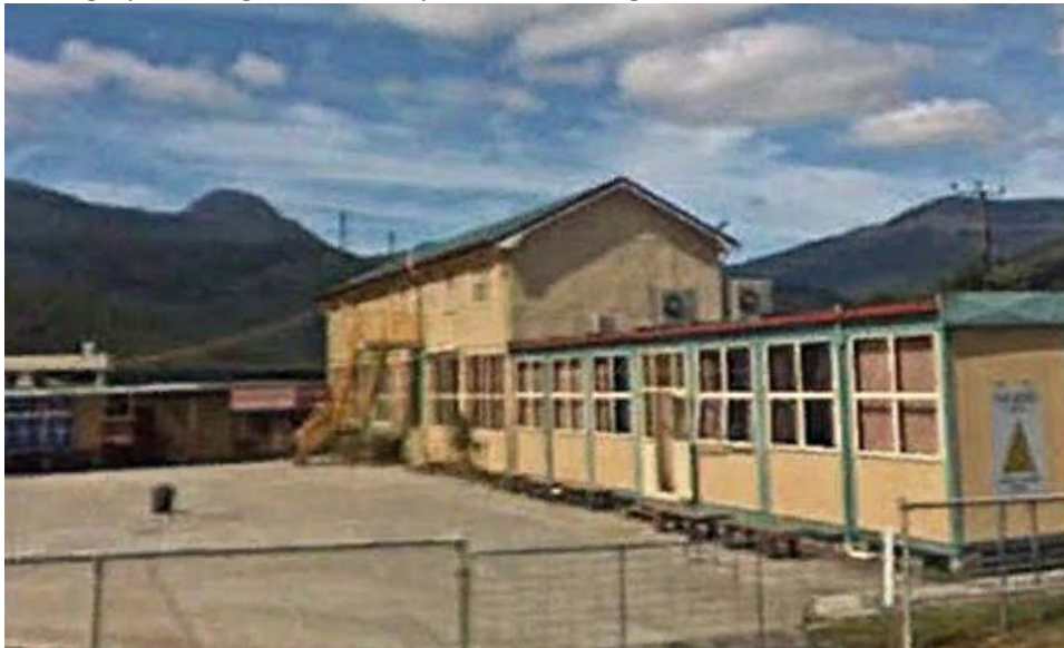
Photograph of original Rosebery School building (frame/timber to be used for shed)
