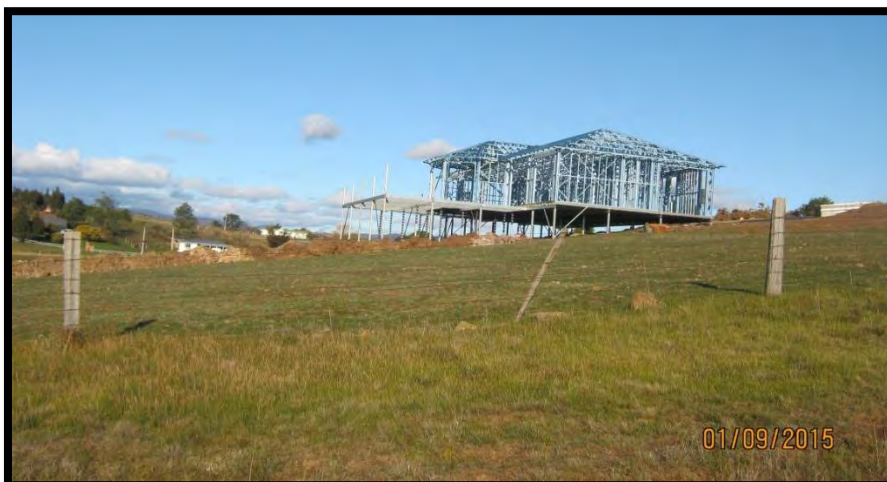
^New dwelling under construction at 31 Park Street, approximately 100m north of the proposed dwelling site (65m from northern boundary of subject site).
