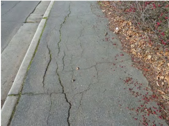
293 Footpath damage caused by Tree roots or sub grade conditions
