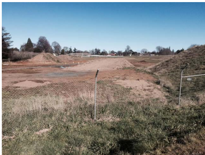
The Borrow Pit
