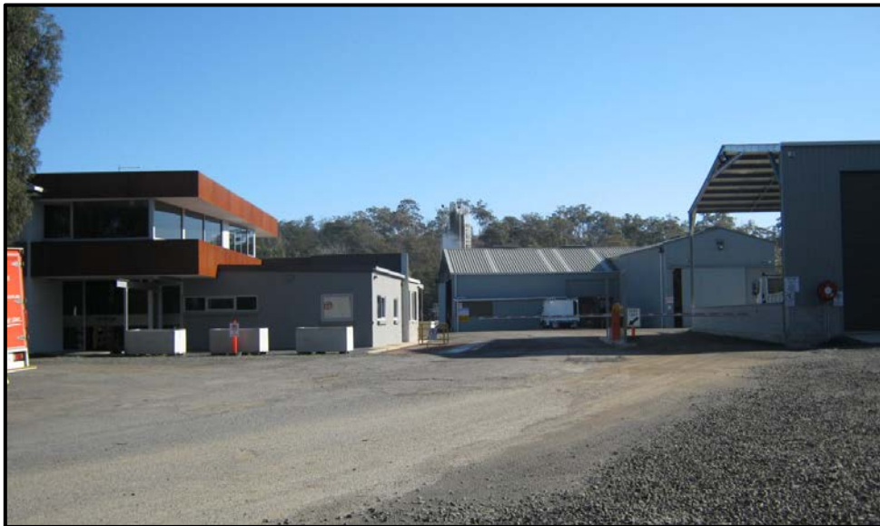
Figure 2 – existing buildings on Digga Excavation site
