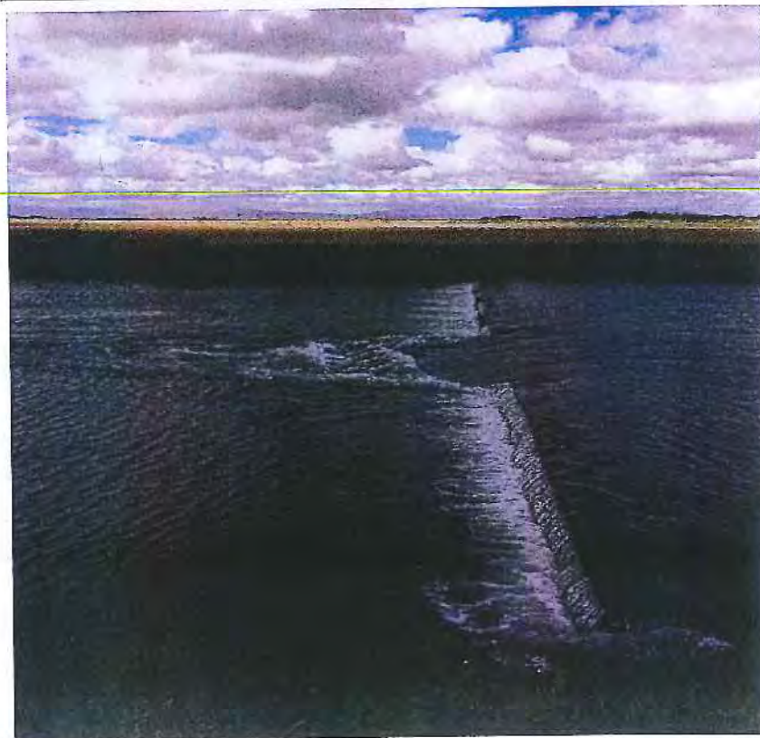
The weir on Brumby's Creek
