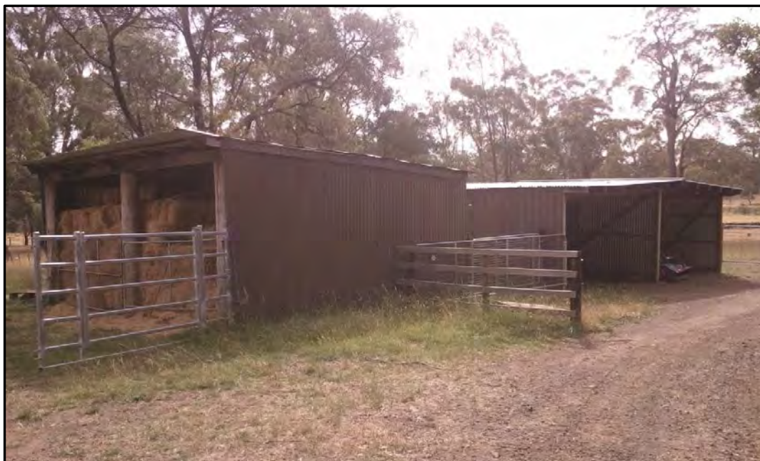
Figure 1 – sheds to be removed
