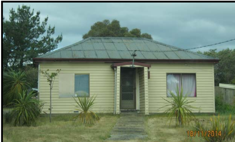
^Existing dwelling on site to be demolished.
